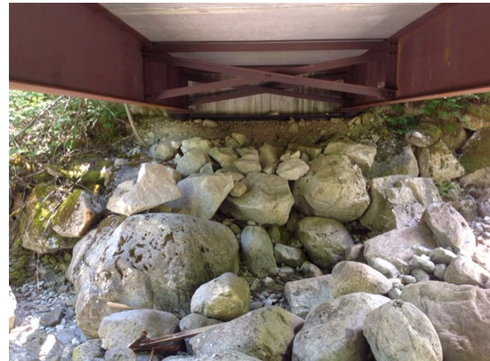
Right Bank Abutment when facing downstream
