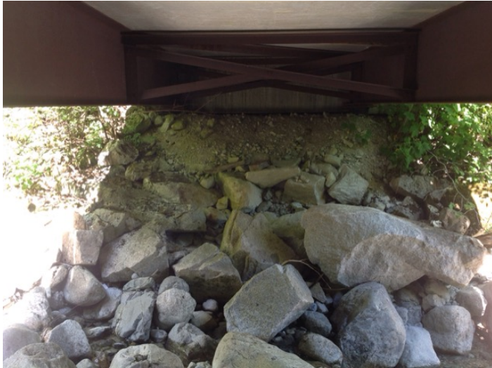
Left Bank Abutment when facing downstream
